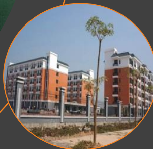
1 st Session Dormitory Building
